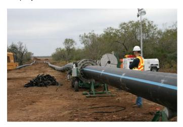
"Quality control and on-site testing were important issues for SAWS," said Radoszewski, "and would have been very costly to do for coated steel pipe. HDPE proved to be a leak-free material, with no cathodic protection required, leading to lower maintenance costs,
